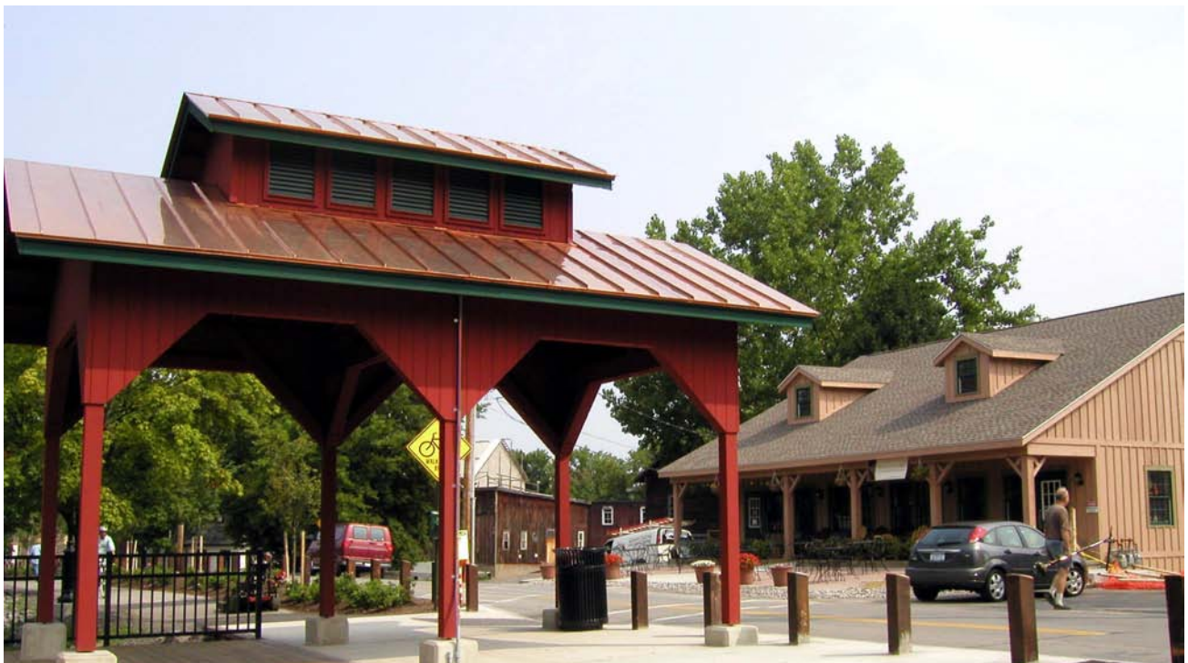
Interpretive gateway pavilion designed by Trowbridge & Wolf. The pavilion, which recalls Schoen Place's history as a canal port, serves as a venue for small gatherings and bands, attracting visitors to nearby businesses.
